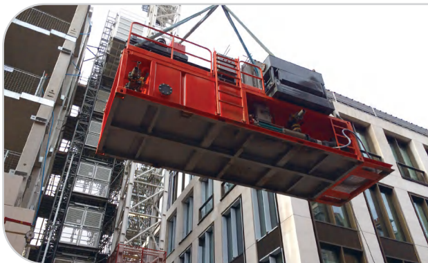
Geothermal Well Drilling Mud Cleaning
